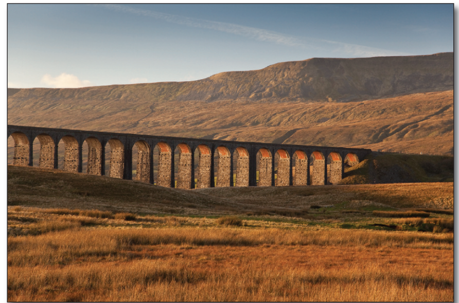
Late afternoon sunshine illuminates the Ribbleshead Viaduct.
